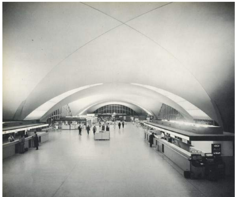
5. The St. Louis Air Terminal: Hellmuth, Yamasaki, and Leinweber, architects. Skylights at the junction points of the interlocking vaults provide natural light, while artificial lighting is placed above eye level. Light is projected upward at the surface of the vaulting, which becomes luminous in gradations.
