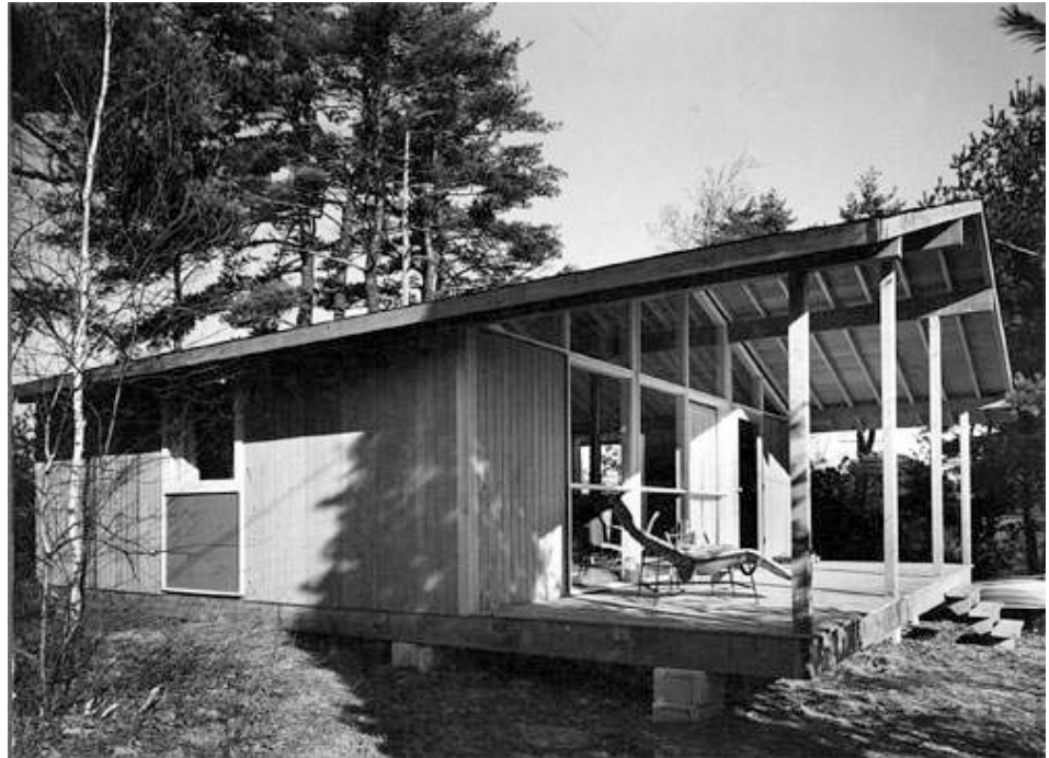
TechBuilt house, circa 1953.
